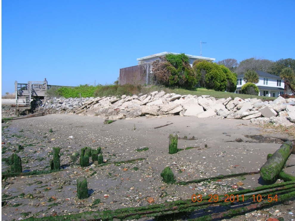
Figure 4.09 March 2011 photo Showing the Eroded Condition and recently added Concrete Rubble at the Southport Pump Station
