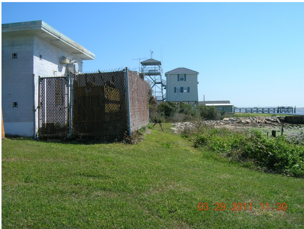
Figure 4.10 March 2011 Photo Showing the Proximity of the Eroded Bank to the Southport Pump Station
