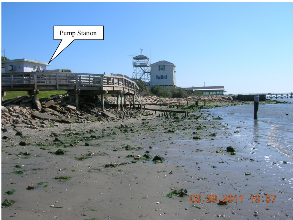
Figure 4.08 March 2011 Photo Looking Eastward along the Eroding Shoreline at Southport Pump Station
