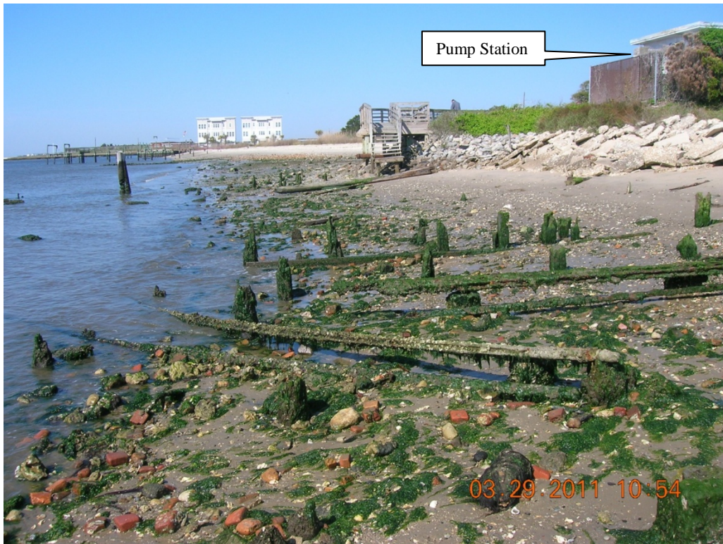
Figure 4.07 March 2011 Photo at Low Tide Looking Westward along the Eroding Shoreline at Southport Pump Station
