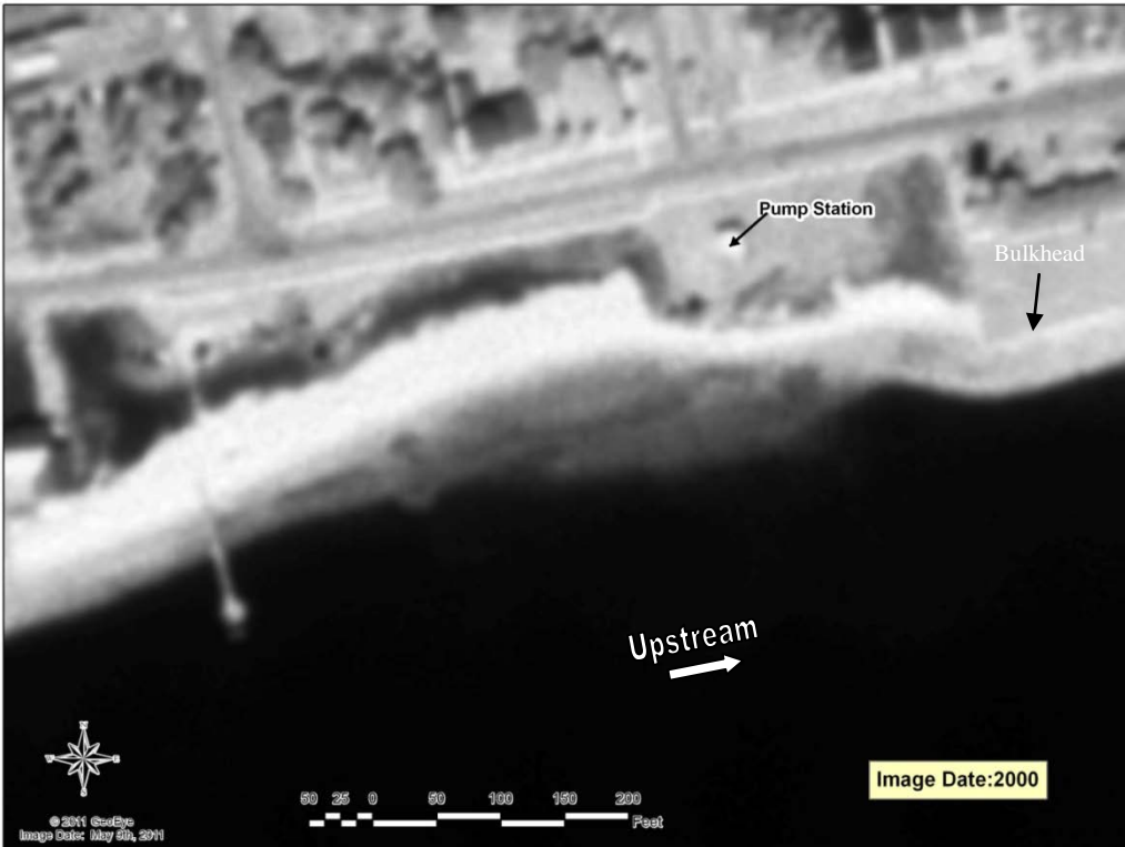
Figure 4.02 Aerial Photograph of Southport Pump Station and Vicinity 2000
