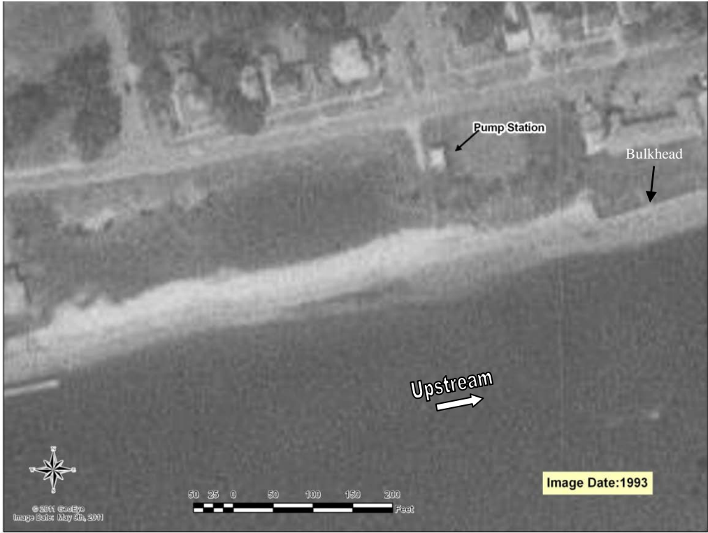
Figure 4.01 Aerial Photograph of Southport Pump Station and Vicinity 1993
